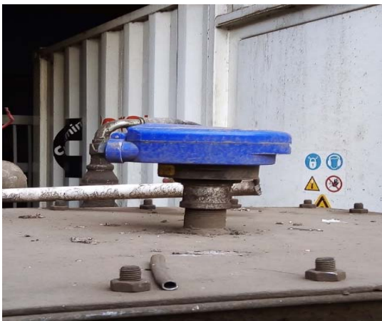
Ultrasonic sensor to monitor fuel level in the generator tanks.
