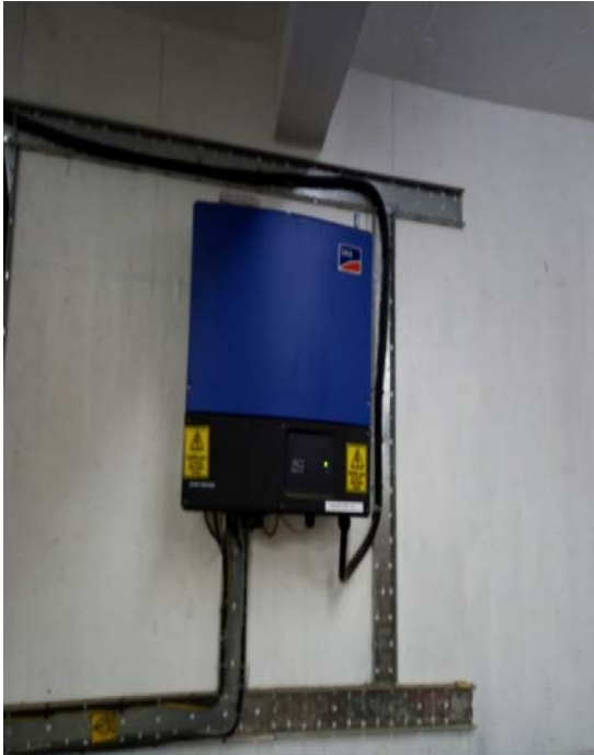
Solar power smart inverters that convert direct current to alternating current for consumption by the building lifts & lights
