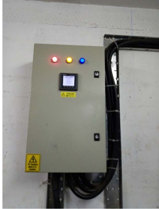
Smart solar meter that monitors real time power production
