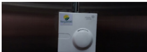
Occupancy sensor that monitors occupation of a room for a maximum of 15min to automatically turn the lights on or off.
