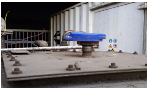
Ultrasonic sensor to monitor fuel level in the generator tanks.
